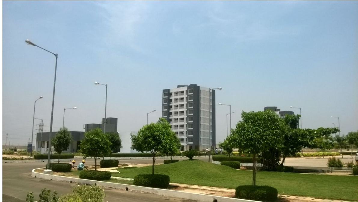
Staff Residential Township Client : L&T Shipbuilding Pvt Ltd
