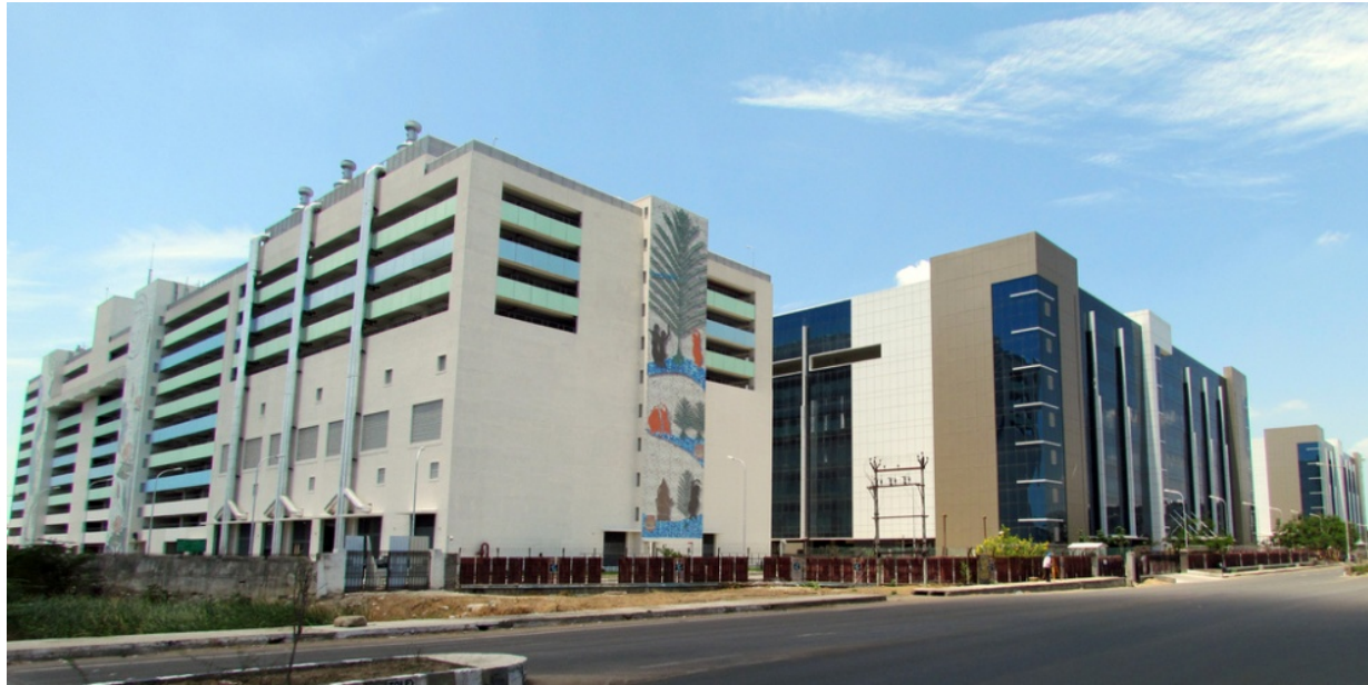
CTS IT FACILITY Client : L&T ECC
