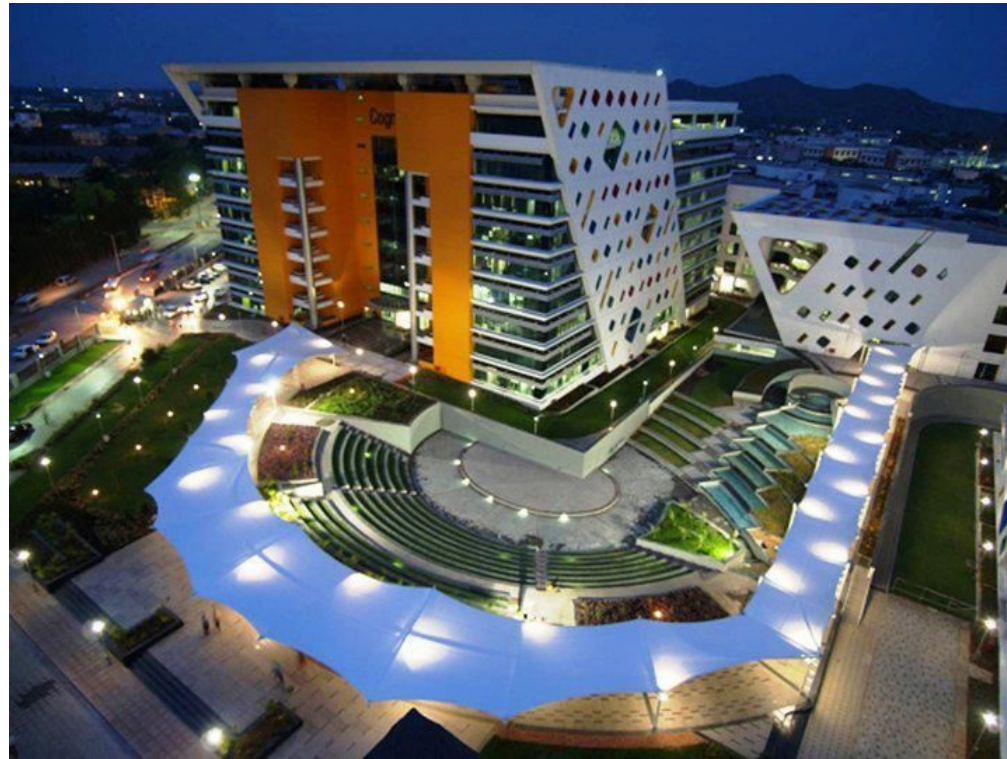
CTS IT FACILITY
