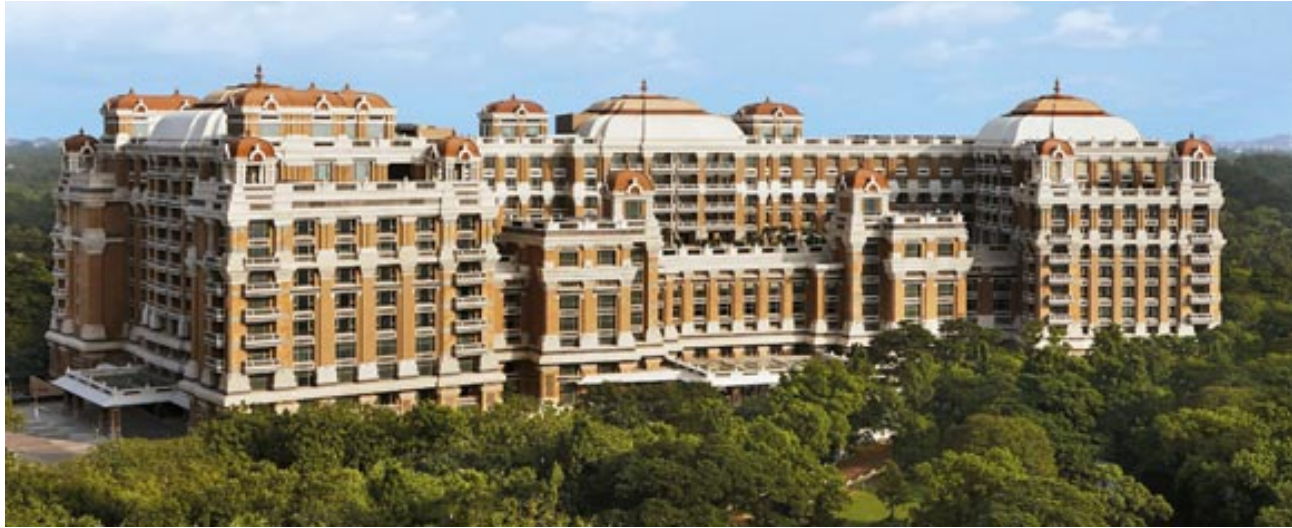
ITC Grand Chola Hotel Client : L&T ECC ltd
