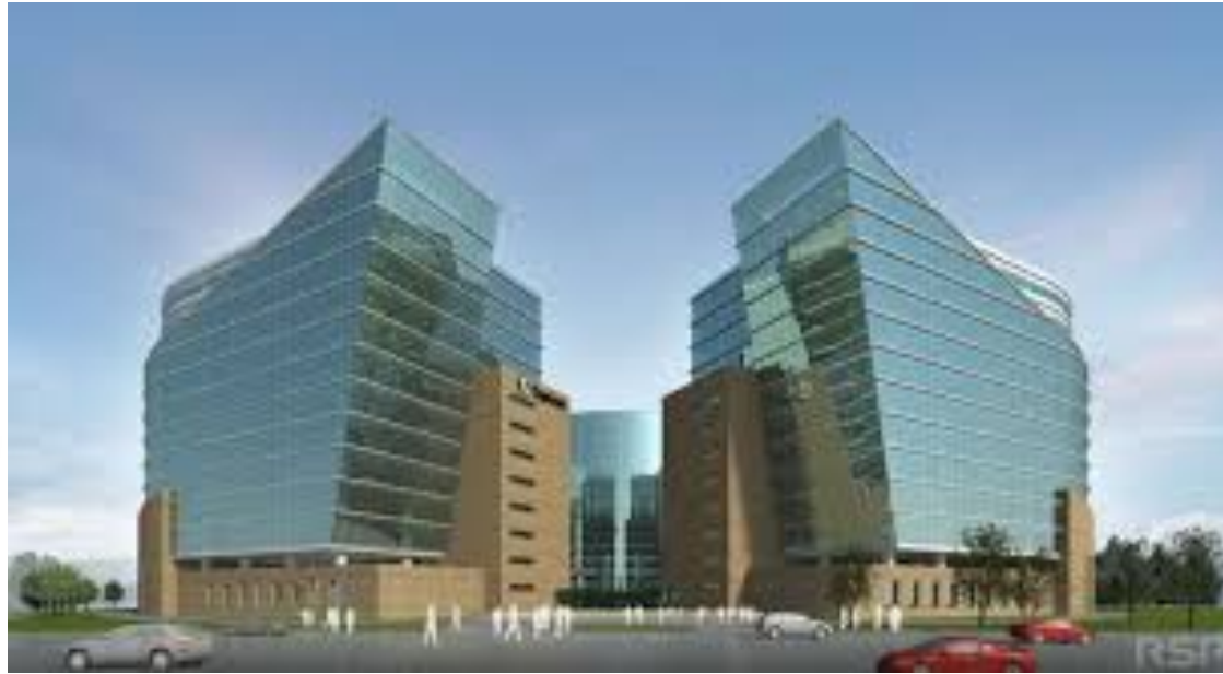
CTS IT FACILITY Client : L&T ECC
